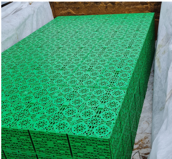
Completed Tank Construction
