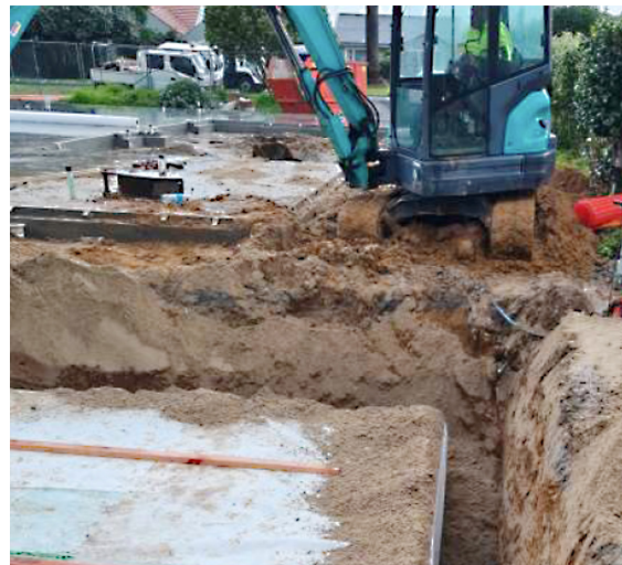
Wrapped Tanks & Back-Filling
