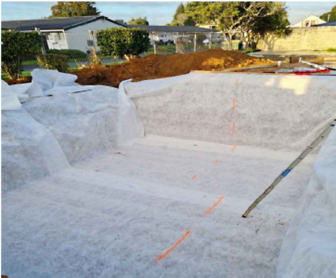
Geotextile Fabric Placement
